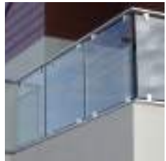
I: METAL FRAM HANDRAIL WITH GLASS PANELS
